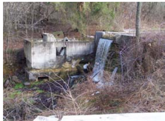
Note the upper and lower water spill release
